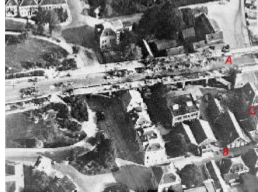
Picture of the bridge shortly after the first attempt by SS recon forces to take it. The large number of burnt out vehicles and wreckage can clearly be seen.
